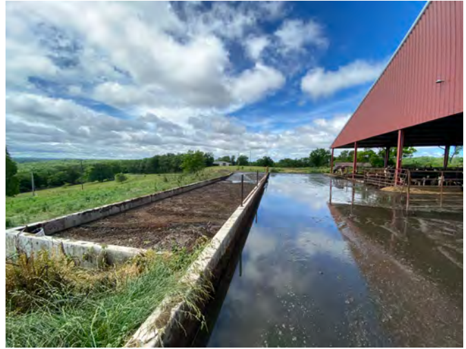
Figure 7c. PPSB and sand lane in operation.
