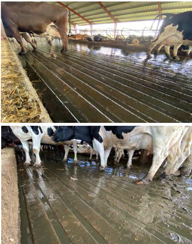
Figure 6a and 6b. Upslope (top) and downslope (bottom) of flush alley.
