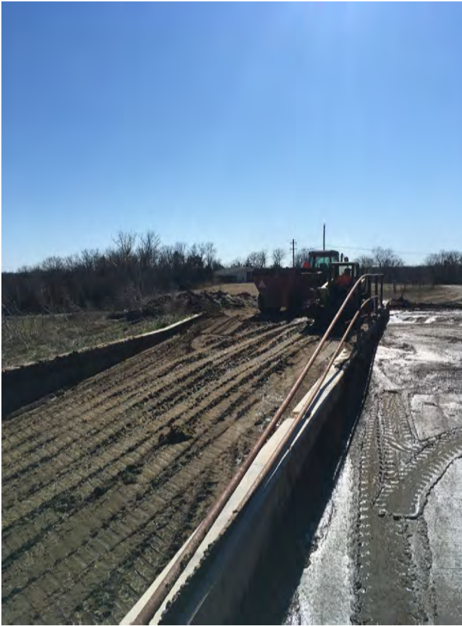
Figure 7b. PPSB ramp and adjoining sand lane.
