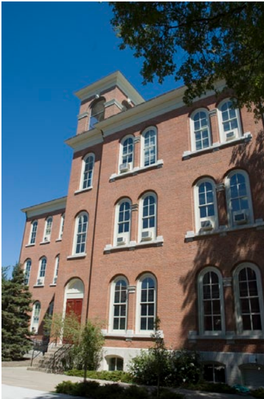
Side view of Switzler Hall, 2005.
