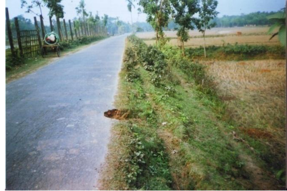
Fig. 4. The raised roadsides having no plantation is also being damaged due to formation of a hole and narrow ditch by rain water. This might cause the accident and damage of vehicles and lives which can be saved following ‘RAMPT’ plantation model as suggested by Hossain (2007).
