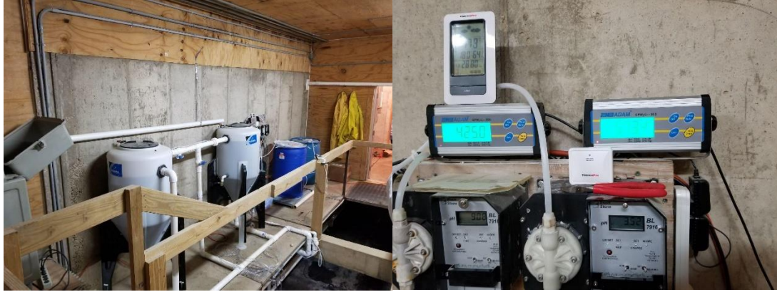
Figure 3. Initial setup of the acid and product tank, acid and base pump, and supplies
