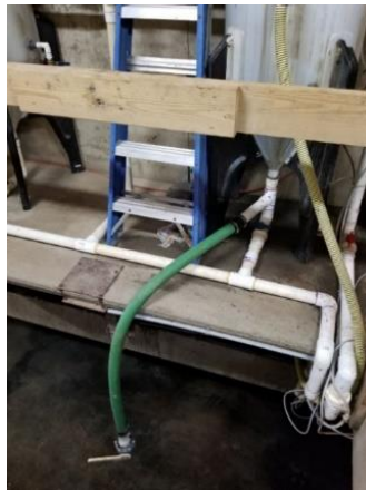
Figure 16. Manual settlement discharge line installed below the acid tank, June 19.
