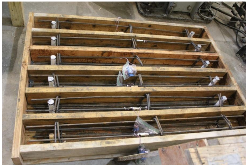
Formwork with the reinforcement of beams (series II).
