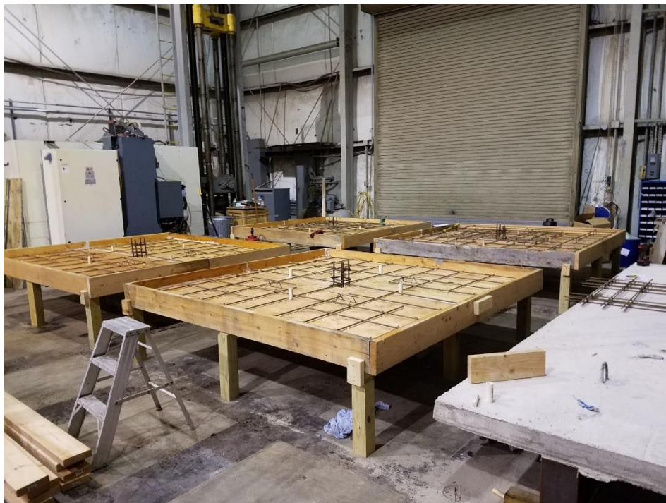
Pad footing with column reinforcement.
