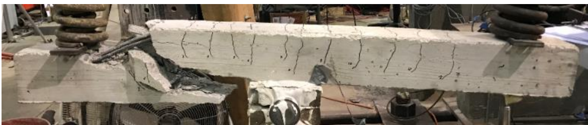
Figure 3-53. Beam 9 (B9-SL) failure.
