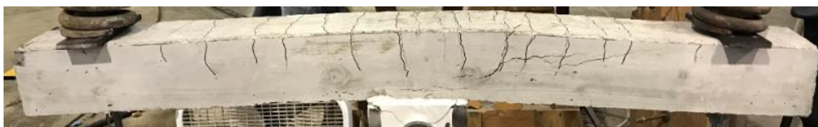
Figure 3-44. Beam 6 (B6-SL) failure.
