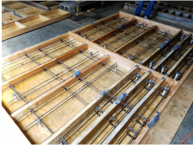
Formworks with the reinforcement of beams (series I).
