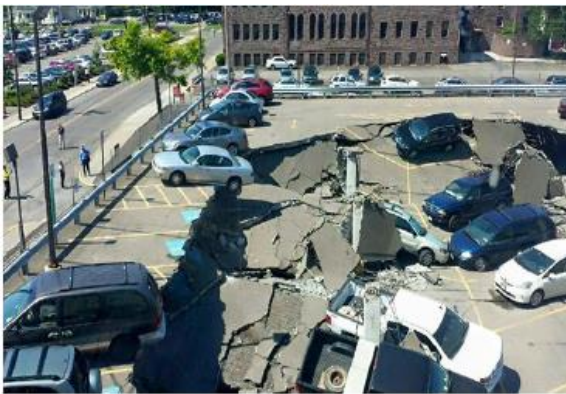
(a) Wilson Hospital parking garage
