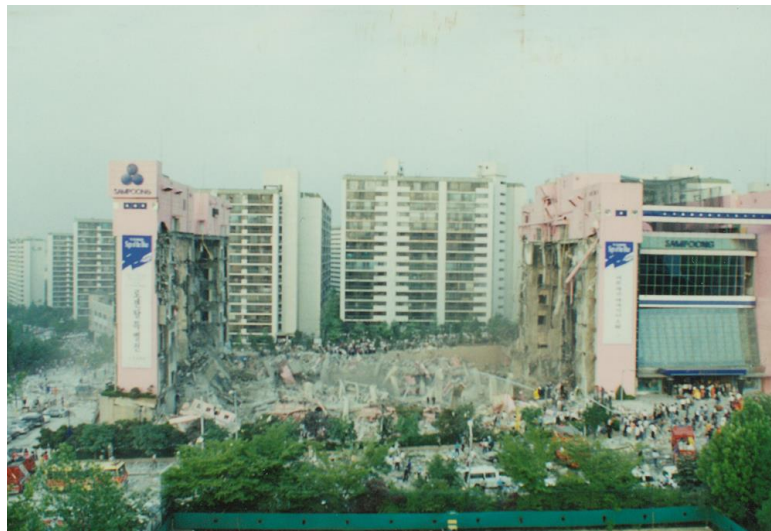
Figure 2-2. North wing collapse of Sampoong Department Store.
