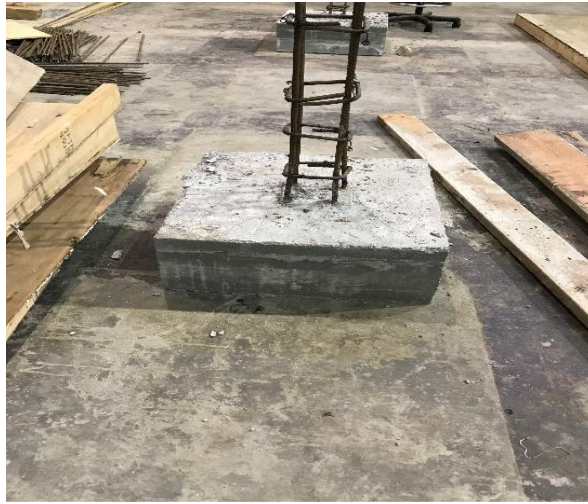
Pad footing with column reinforcement.
