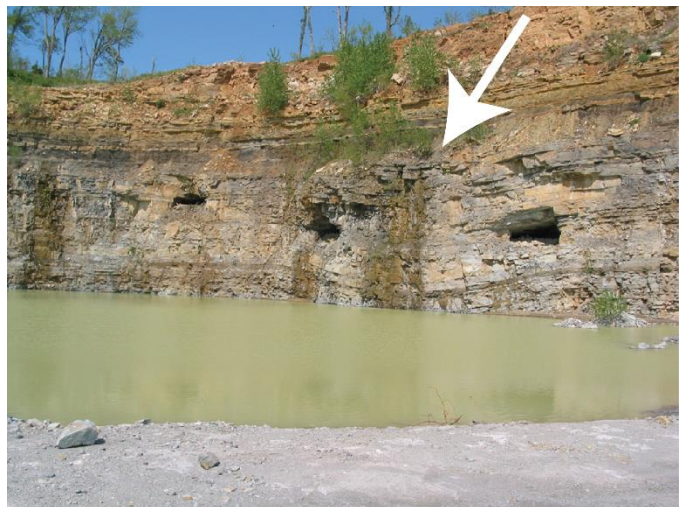
Figure 3-16. Slumping due to limestone dissolution associated with a fluorite ore body at the Hastie Quarry. Adits mark the approximate lateral extent of the ore body. Photograph credit: Martin Appold
