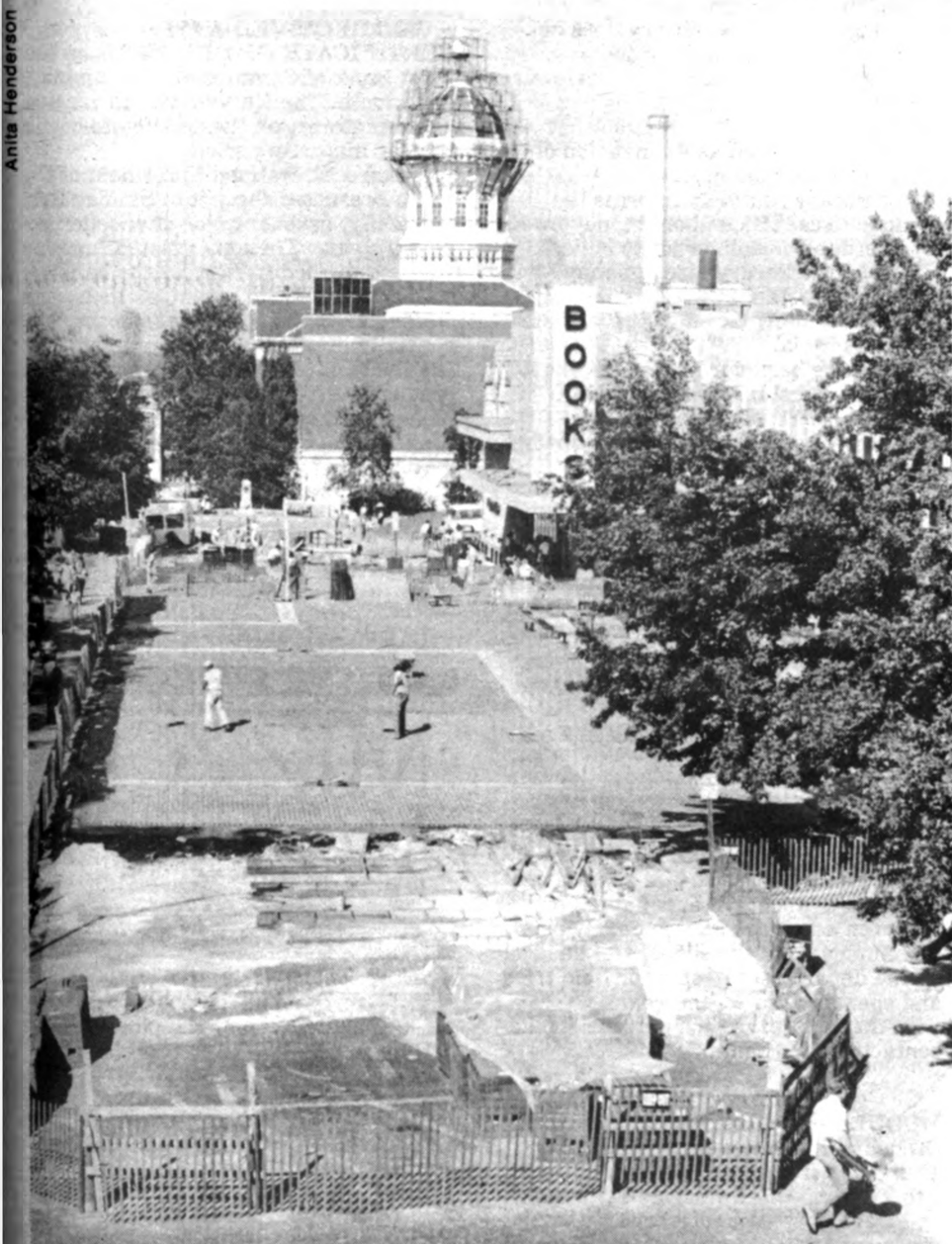
Construction on Lowry Mall, as viewed from Memorial Union.
