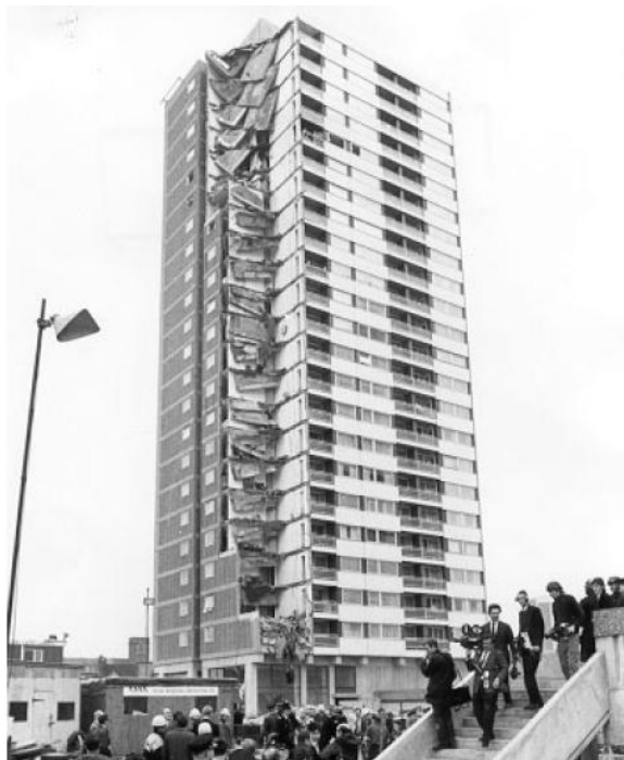
Figure 2-1. Ronan Point building after collapse (Nair, 2004)
