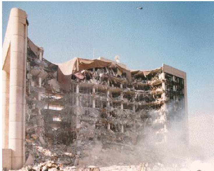
Figure 2-2. Murrah Federal Office Building after 19 April 1995 attack (Crawford, 2002)
