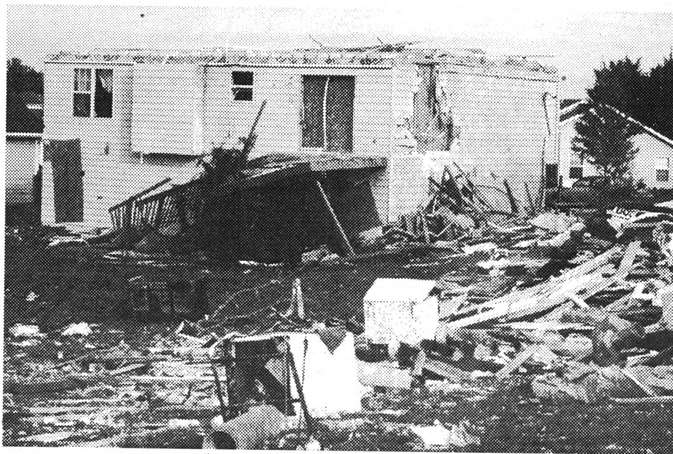
Matt and Renette Reiske had to rebuild their Columbia home from the ground up after it was ripped apart last fall by a tornado. Help from the Red Cross, a United Way agency, made their burden lighter.
