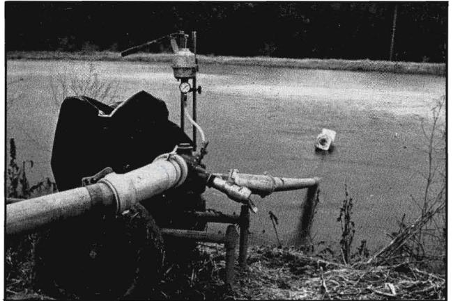
Figure 11. A pump intake floated 1-2 feet below the surface will be least likely to plug.
