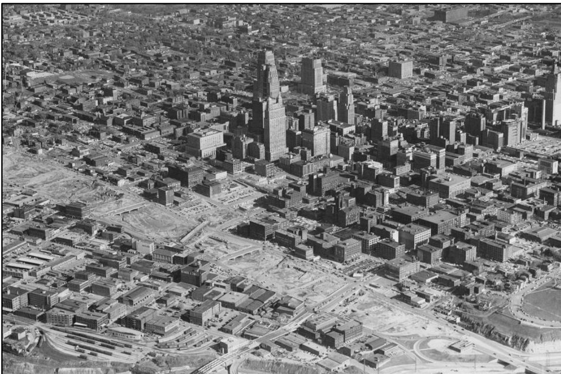
Figure 4.9. Downtown Kansas City, Missouri in 1957, showing the area cleared for the Downtown Loop freeway. Source: “KC Q - Kansas City’s Downtown Loop,” Missouri Valley Special Collections, Kansas City Public Library, Kansas City, Missouri, accessed April 13, 2023, https://kclibrary.org/blog/kc-q-kansas-citys-downtown-loop .
