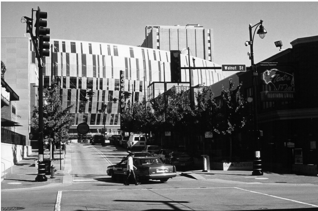
Figure 14. The Sprint Arena across from the Power & Light District in downtown Kansas City.
