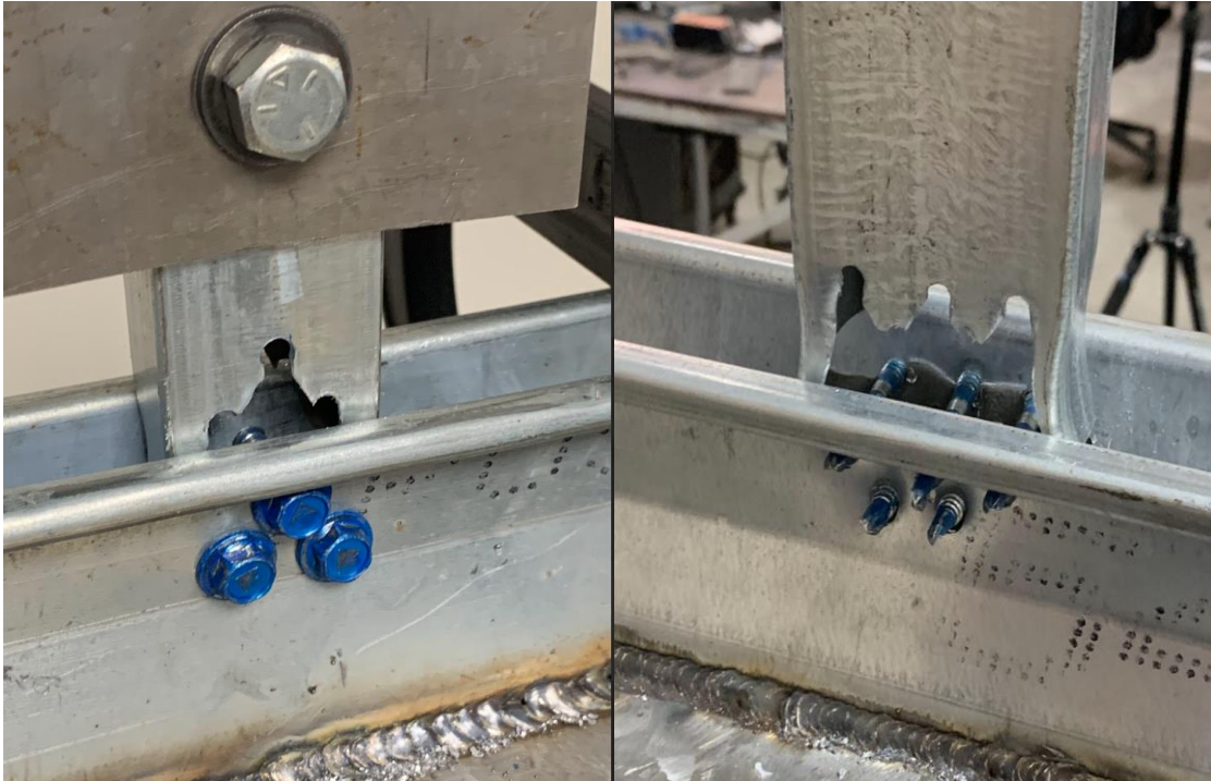
Figure 62: Block Shear Failure
