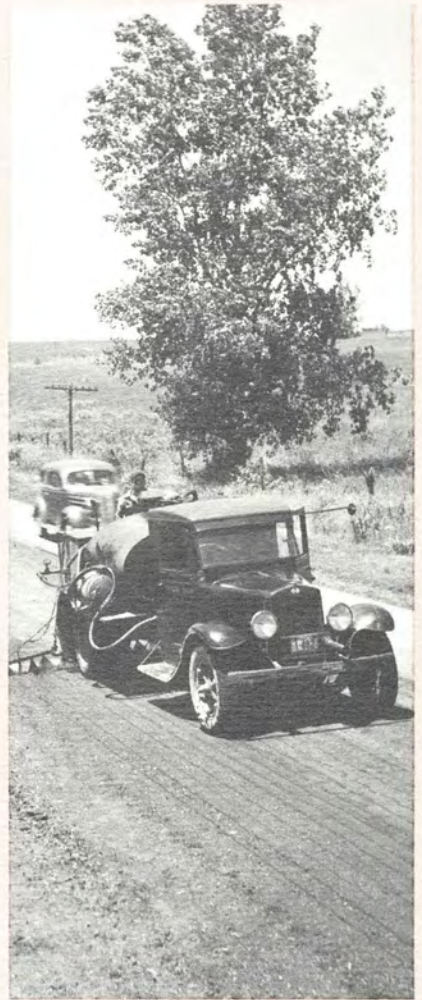
Coming fast, a Missouri motorist of the '30s passes a Highway Department asphalt distributor.
