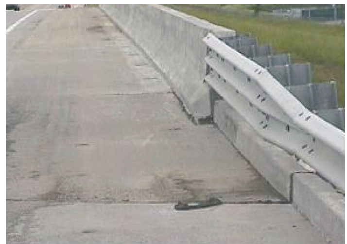
Figure 5 Bridge Approach Slab Observed During Survey
